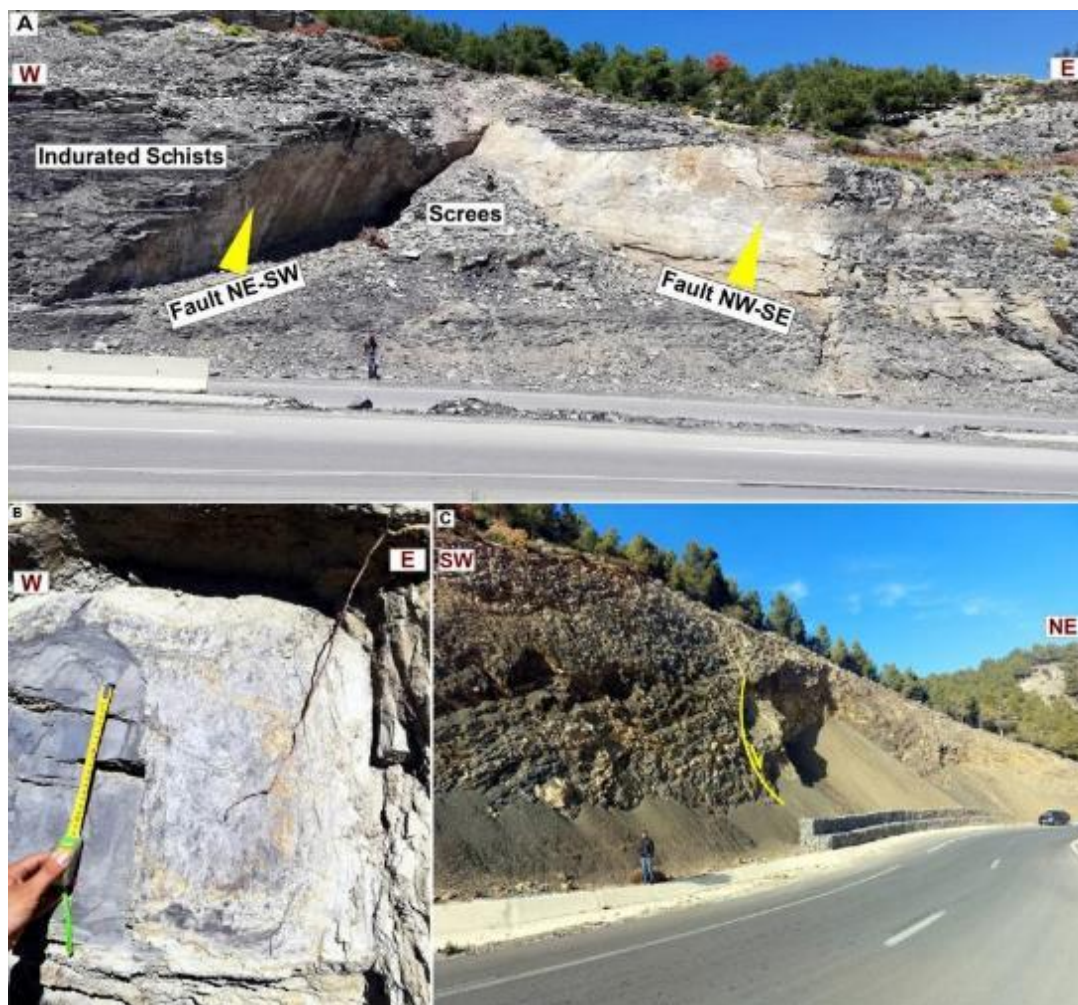
Fig.5. Types of landslides in the study sector. A wedge sliding at the intersection of two fractures (example: intersection of NE-SW and NW-SE faults). B- Planar sliding on stratified surfaces. C- Rotational sliding.
